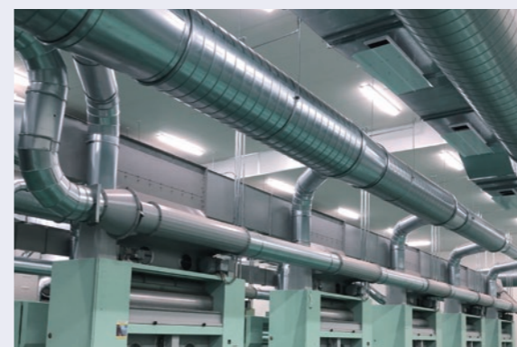
Variation of duct system Cotton-feeding duct, air-transport duct, dust collecting duct, air conditioning duct
